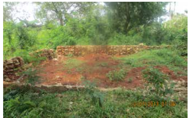
Fig (5.6): Foundation of an abandoned development near Chauringo Quarry.
